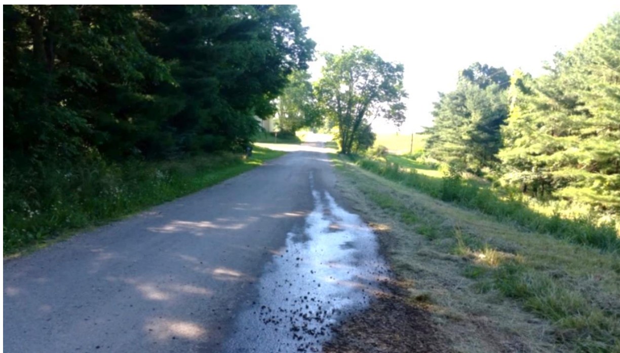
FIGURE 19: OIL & GAS BRINE ON ROAD, GUERNSEY COUNTY
